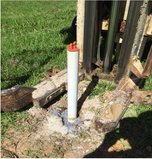
Photo 13: Monitoring Well MW01 prior to backfill
